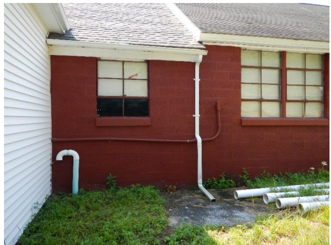
Sanitary vent below window
