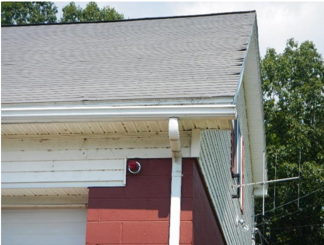
Cupped / unsealed roof shingles
