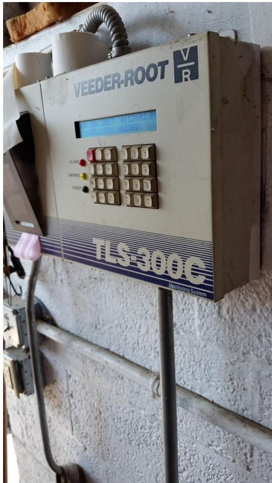
Photo 7.2 Gasoline Tank Monitor Alarm
