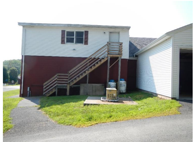
Unprotected exterior Fire Stair Propane tanks (Hazard) under Stair Propane tanks below operable openings (door / window)
