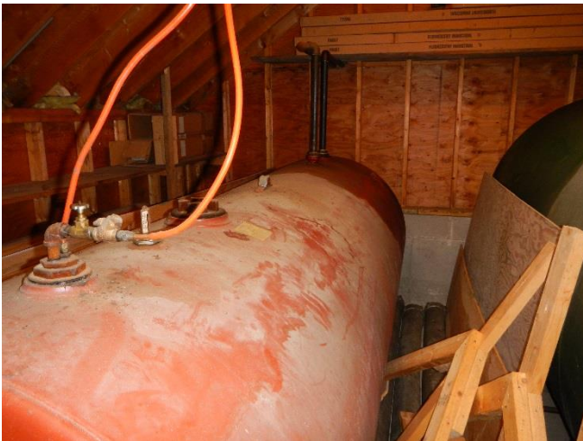
1000 Gal. fuel oil tank Below Police Dept. space Uninsulated exterior walls / roof
