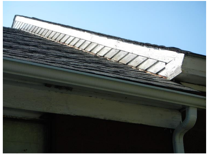
Siding with paint loss / partial deterioration
