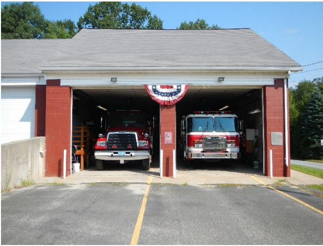
Retaining wall without guardrail Deflection noticeable in ridgeline
