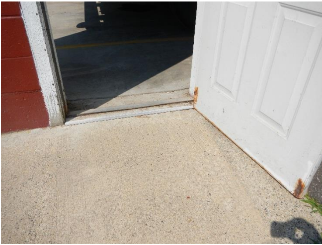
Rust / Deterioration of exterior metal door Deterioration of lower wood door jambs
