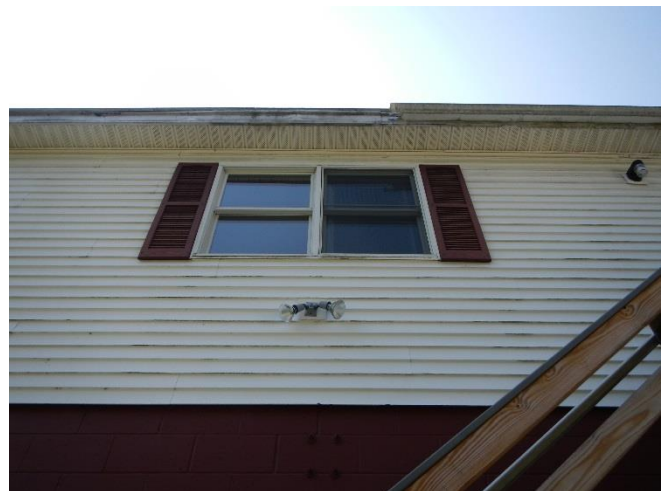
Missing roof gutter section
