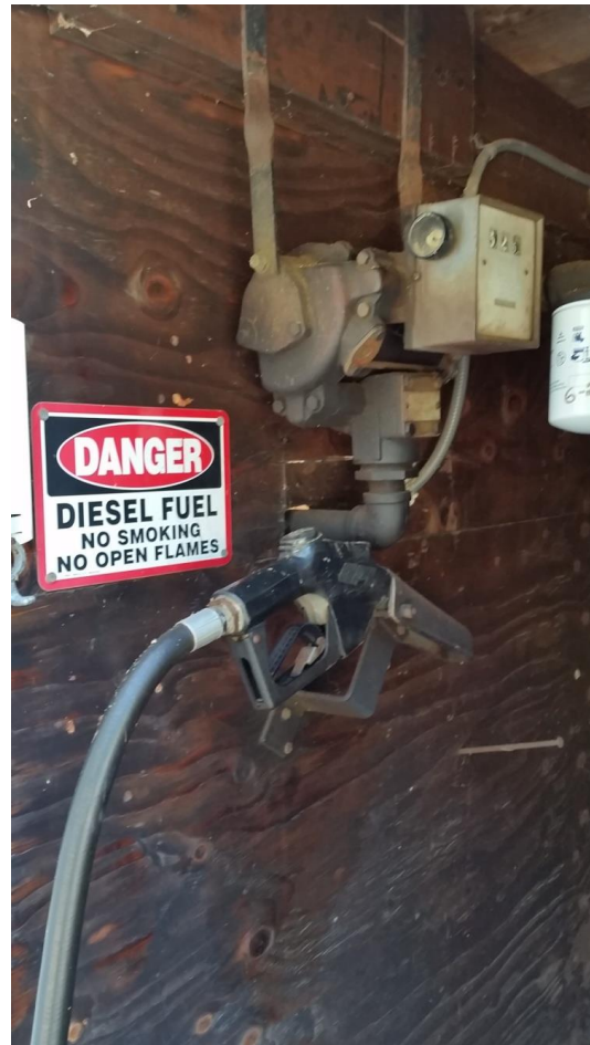
Photo 7.3 Diesel Nozzle
