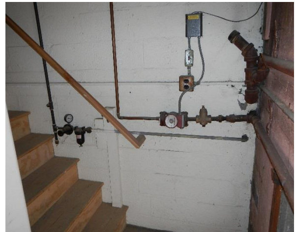
Lower Fire Stair landing Non-compliant Stair Additional utility hazards to emergency egress
