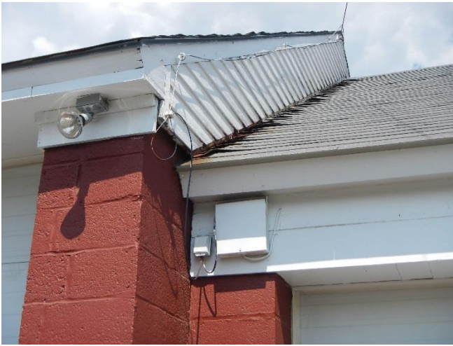
Cupped / unsealed roof shingles
