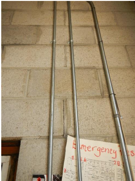
Cracked Concrete Masonry Units (CMU)
