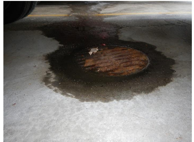
Apparatus Floor Drain Leaches below building
