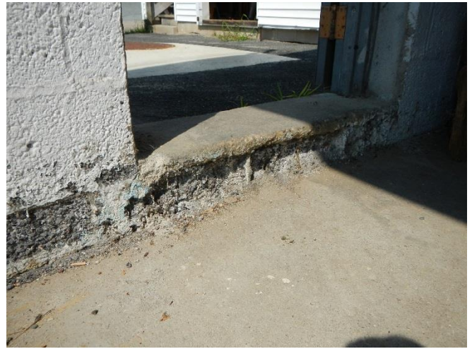
Deteriorate CMU below door threshold
