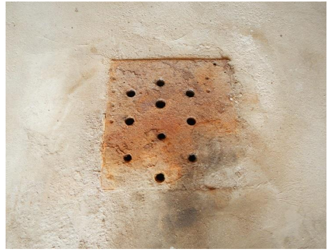
Apparatus Floor Drain Leaches below building
