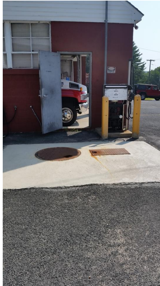
Photo 7.1 Gas pumps & underground tank
