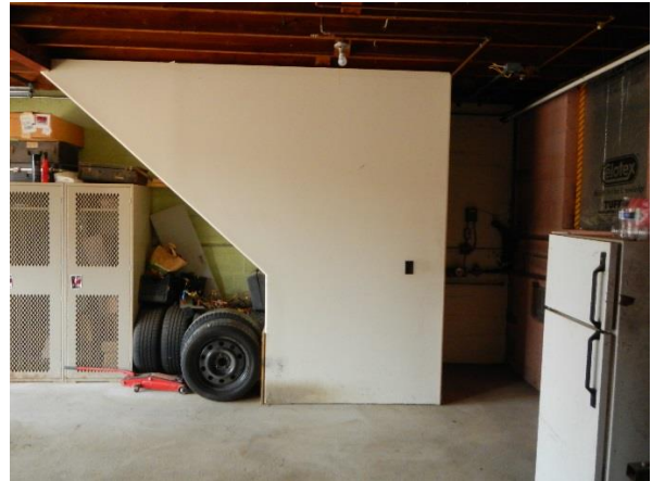
Unprotected Fire Stair discharging into Apparatus bay
