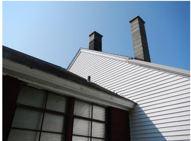
Unfinished / unprotected CMU Chimneys
