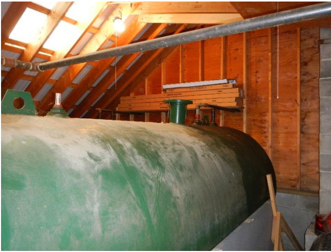
2000 Gal. Diesel fuel tank Below Police Dept. space Uninsulated exterior walls / roof
