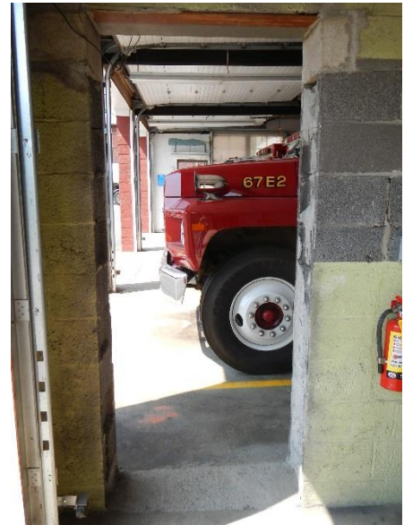
Opening between Apparatus bay additions Cracked CMU joint on left Unprotected primary phone line at upper left
