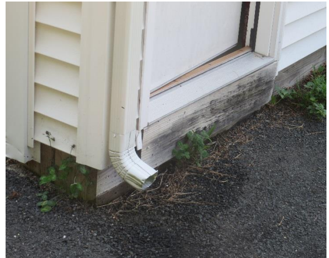
Photograph #8 – 6x6 Wood Sleepers below Exterior Wall
