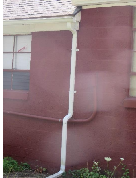
Photograph #6 – Vertical Crack in CMU Wall
