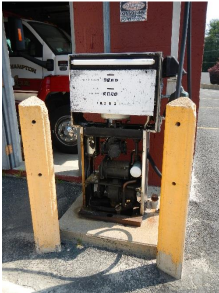
Exposed / Degraded Gas pump
