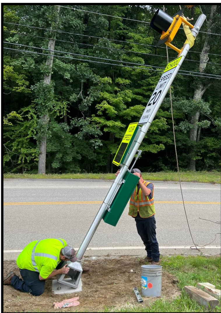
IMAGE: Westhampton Highway Department staff install one of two solar- and battery-powered speed monitoring and feedback signs on Kings Highway near the Westhampton Elementary School.
